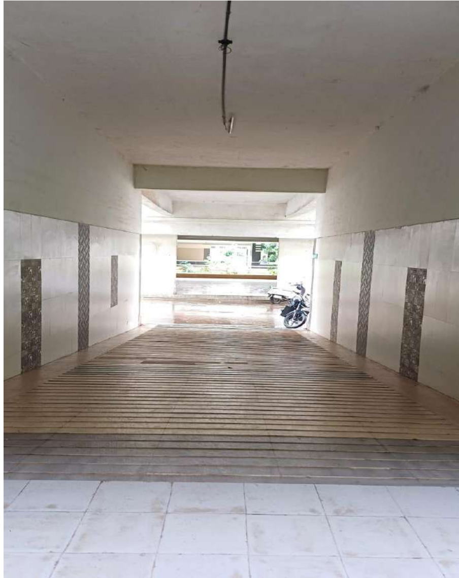
Divyangjan Friendly Ramp
